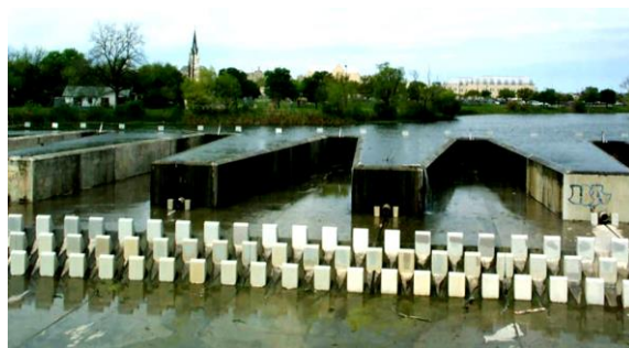
Fig.2- Richard Dam overflow in America
